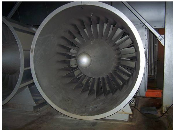
Figure 7. Axial Vane Fan located at the 10x10 SWT.
