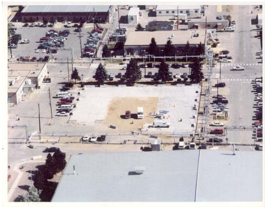
Figure 1. Under Building Contamination 123: the 'U' shaped concrete slab is located in the center of the photograph.
