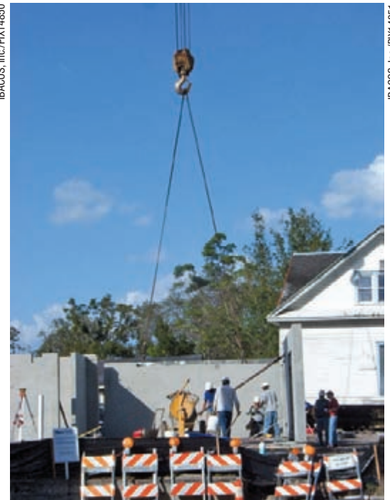
Pre-cast exterior concrete walls allow for faster building enclosure construction and a tighter envelope.
