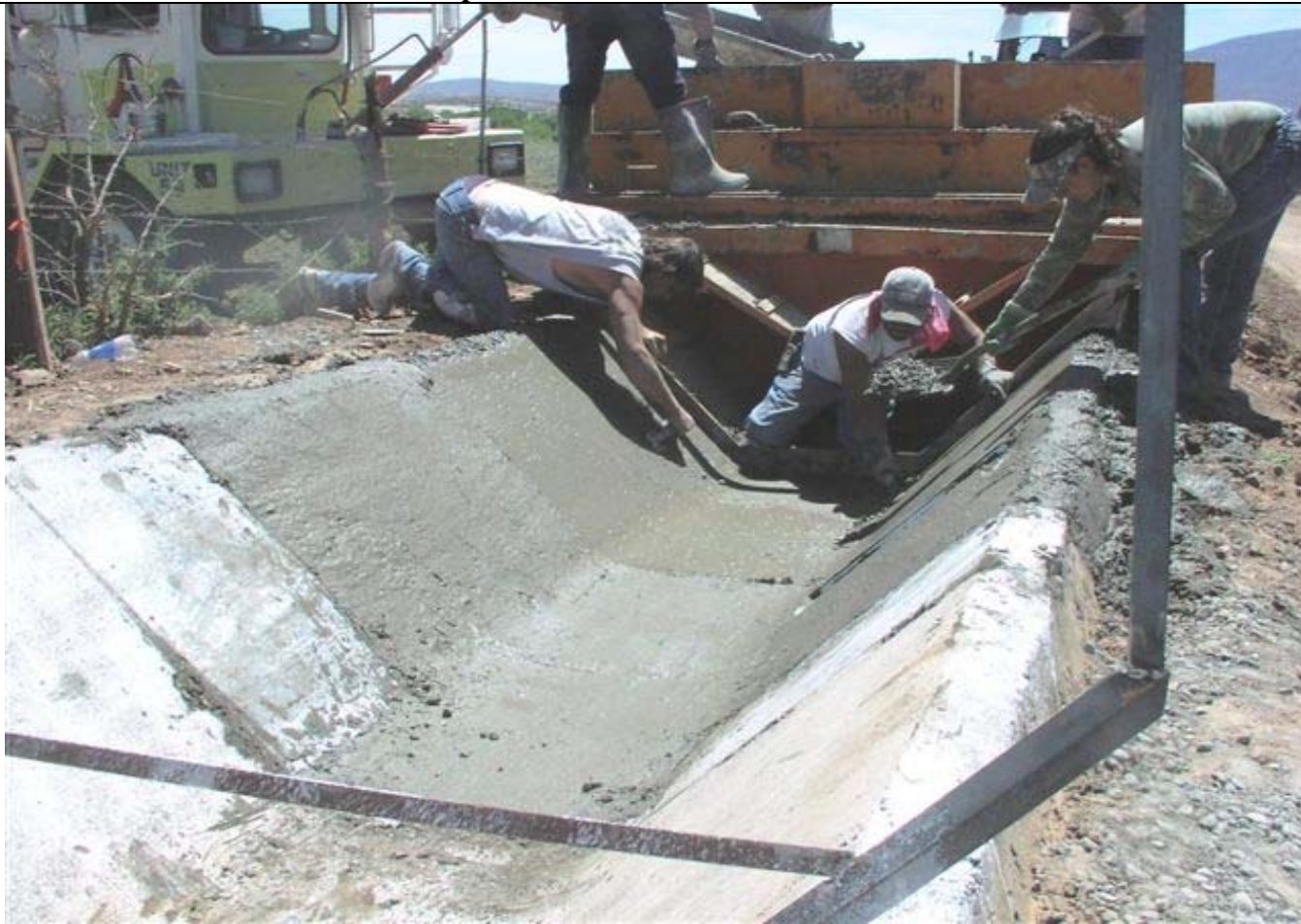
Slip form ditch under construction
