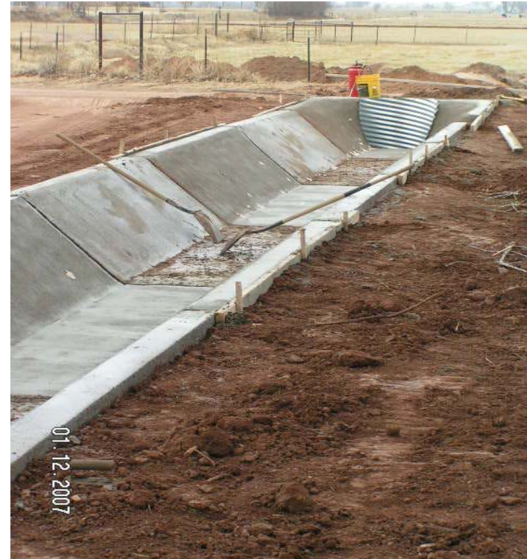
Hand Placed Ditch
