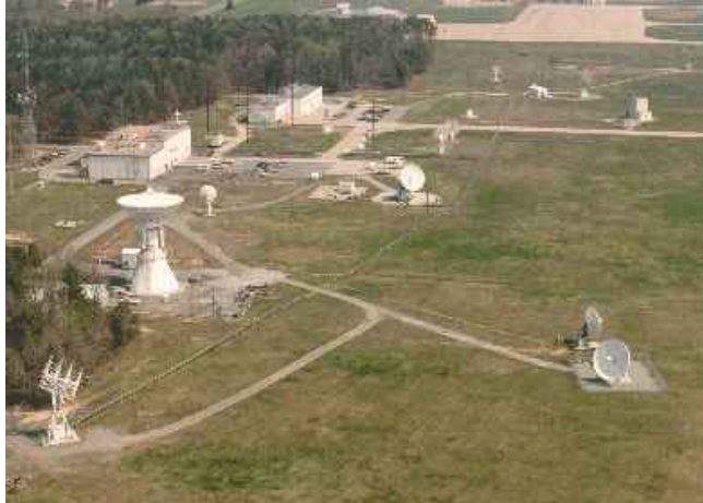
Figure 3-18. Range TM Facility and WOTS
