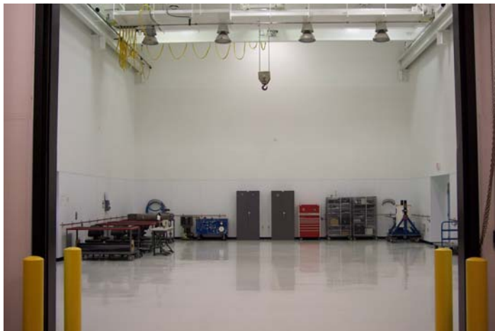
Figure 3-13. 100K Clean Room in MPPF (East High Bay)
