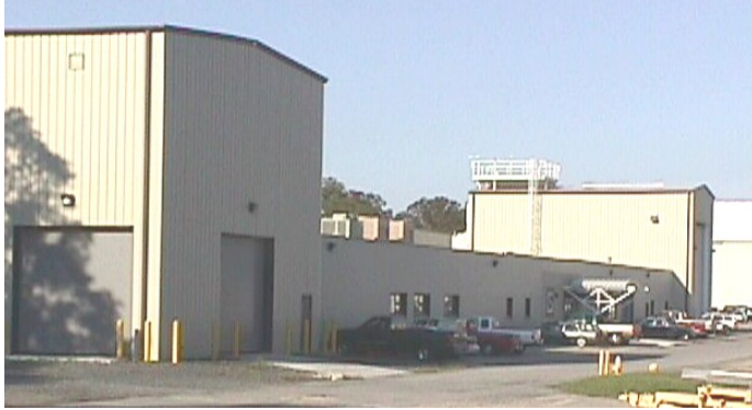
Figure 3-12. Multi-Payload Processing Facility (MPPF/F-7)
