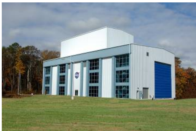
Figure 3-11. Payload Processing Facility (PPF/H-100)
