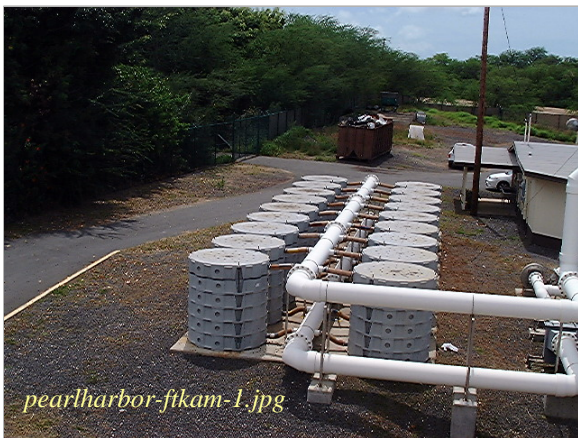
pearlharbor-ftkam-1.jpg Photo: Ft Kam - Odor Control Biotowers Taken By: Greg V. Arthur Date: 04/10/06
