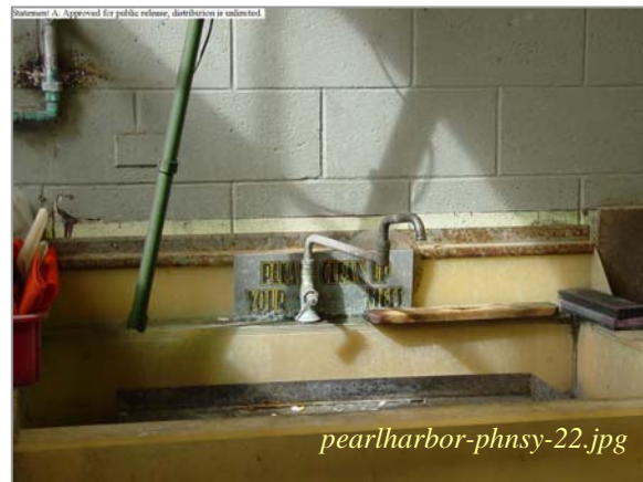
Photos: Bldg 67 - Brushplating Table and Sink Discharge to the 5,000 gal Holding Tank Taken By: Christie Chun, PHNSY Date: 04/12/06
