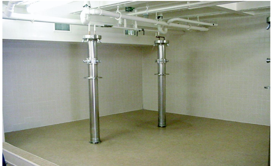
Figure 6: Renovated Showers at Marine Corps Recruit Depot, San Diego
