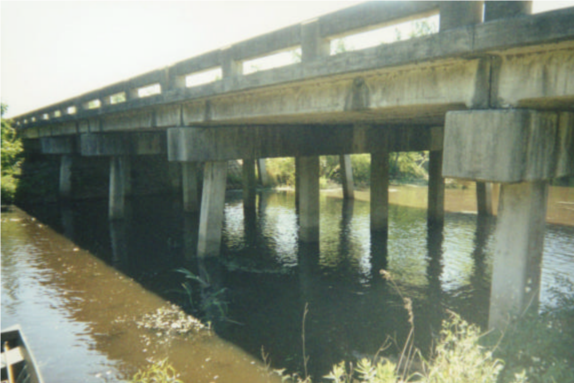
Figure 3-2. The I-10 bridge at Hope Canal.
