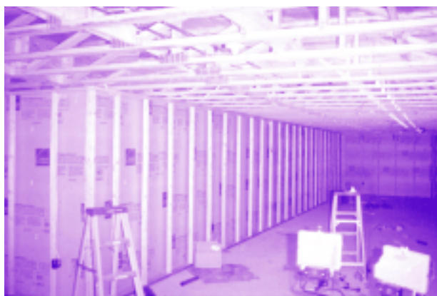
Rigid insulation can be installed in basements above concrete floor slabs and coupled with a floating floor
