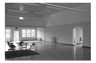
The Auditorium was opened up to the south porch (seen on the left of the photo) and the west wall doorways were filled in (seen on the right of the photo. The collar ties can be seen at the top of the photo.
