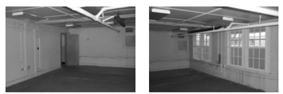
Basement Billiard Hall room shows columns engulfed by the partition wall. Surface mounted conduit and plumbing run helter-skelter throughout. The windows open onto a generous light well but are currently covered with security grating.
