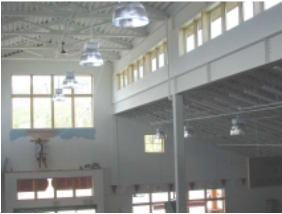
Figure 4. South Clerestory Windows
