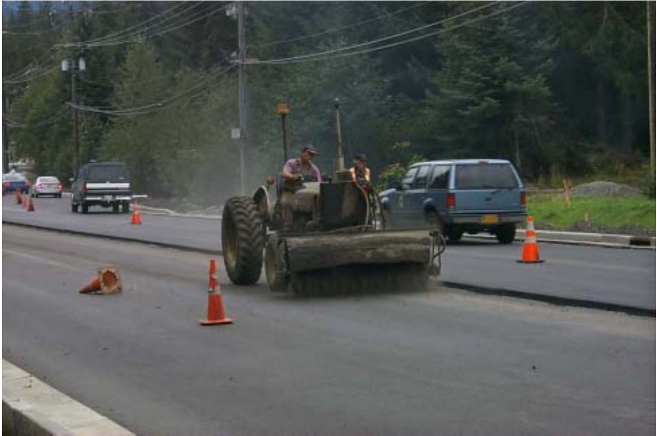
Figure 5-1 Power brooming before tacking
