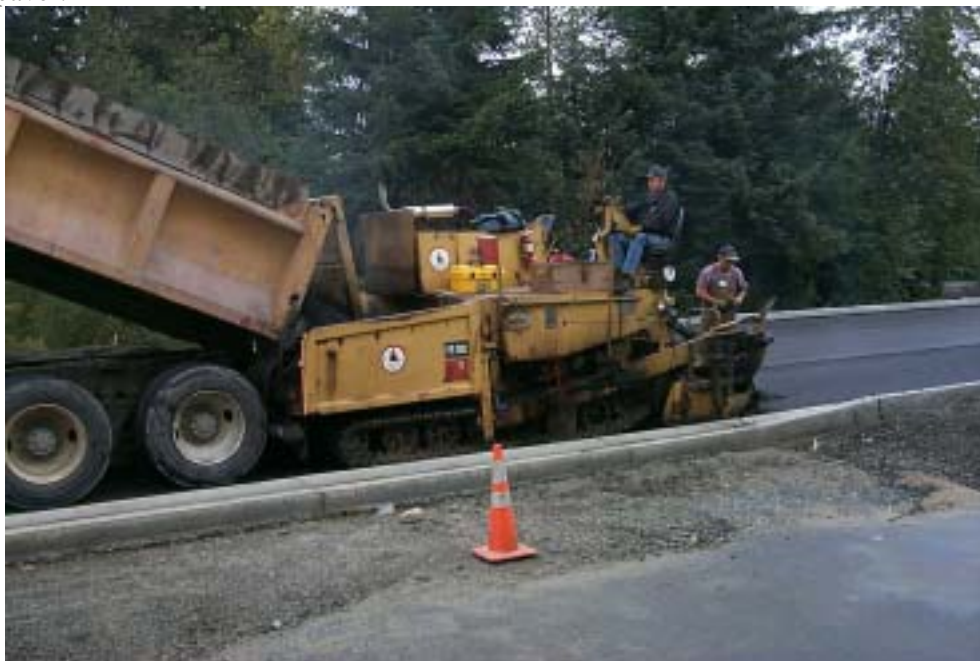
Figure 6-8 Paver in Operation
