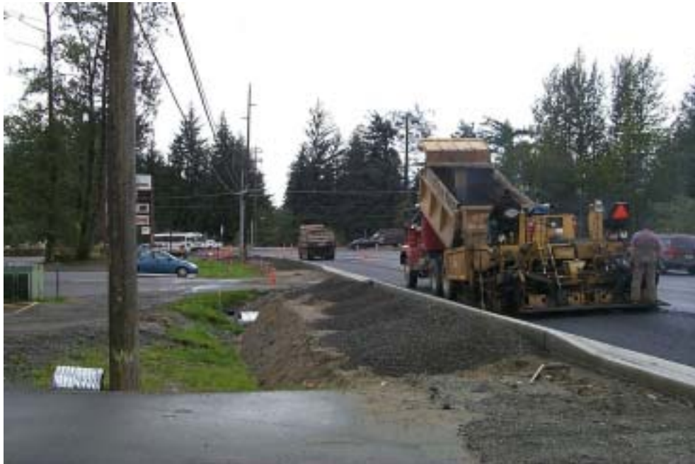
Figure 6-1 Truck Dumping into Paver
