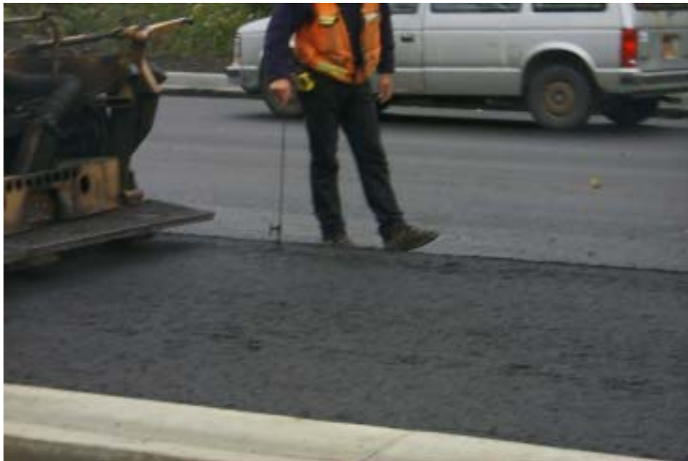
Figure 6-4 Checking pavement thickness
