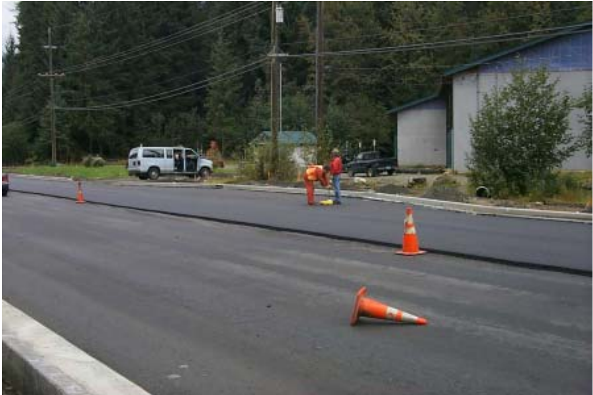
Figure 3-3 Density Testing with a Nuclear Gauge
