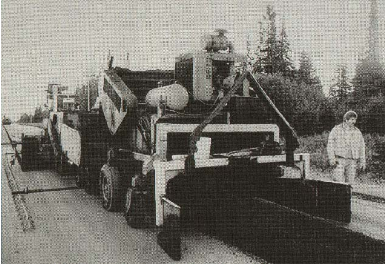
Figure 6-5 Pickup Machine and Paver
