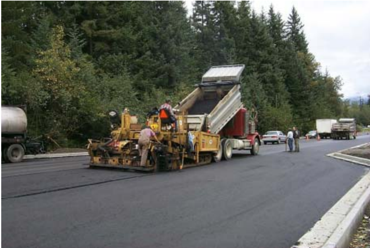
Figure 1-1 Typical Paving Operation
