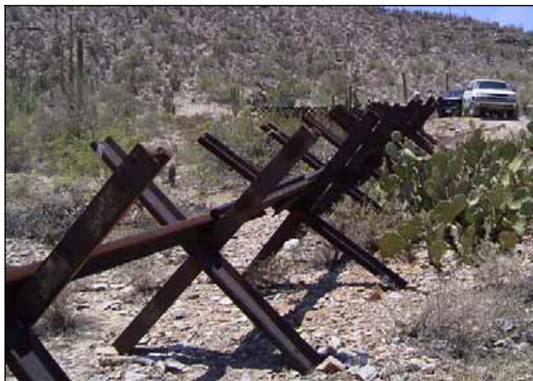
Figure 1-3. Vehicle Fence Type-2 (VF-2)
