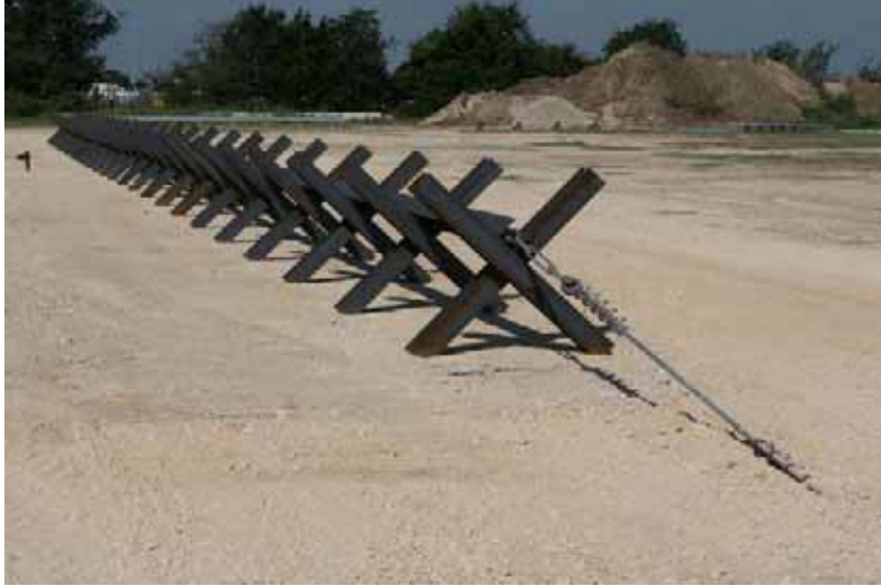
Photograph 2-1. Example of Normandy Style Vehicle Fence
