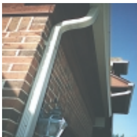
Gutters and downspouts
