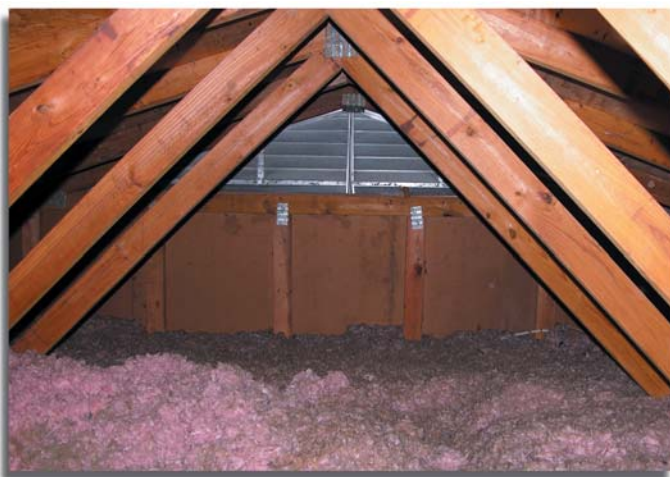
Attics need to be properly sealed and insulated against air exchange and heat exchange between indoors and outdoors. Attic ventilation protects against ice dams.
