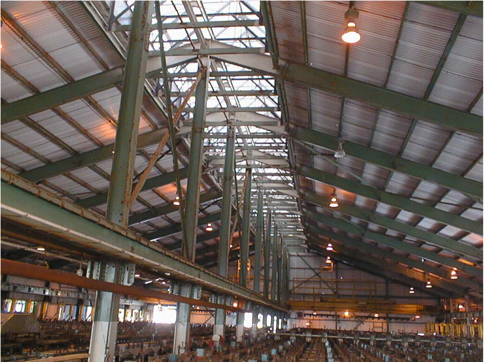
Figure 3-3a. Cell building showing interior of roof ventilator.
