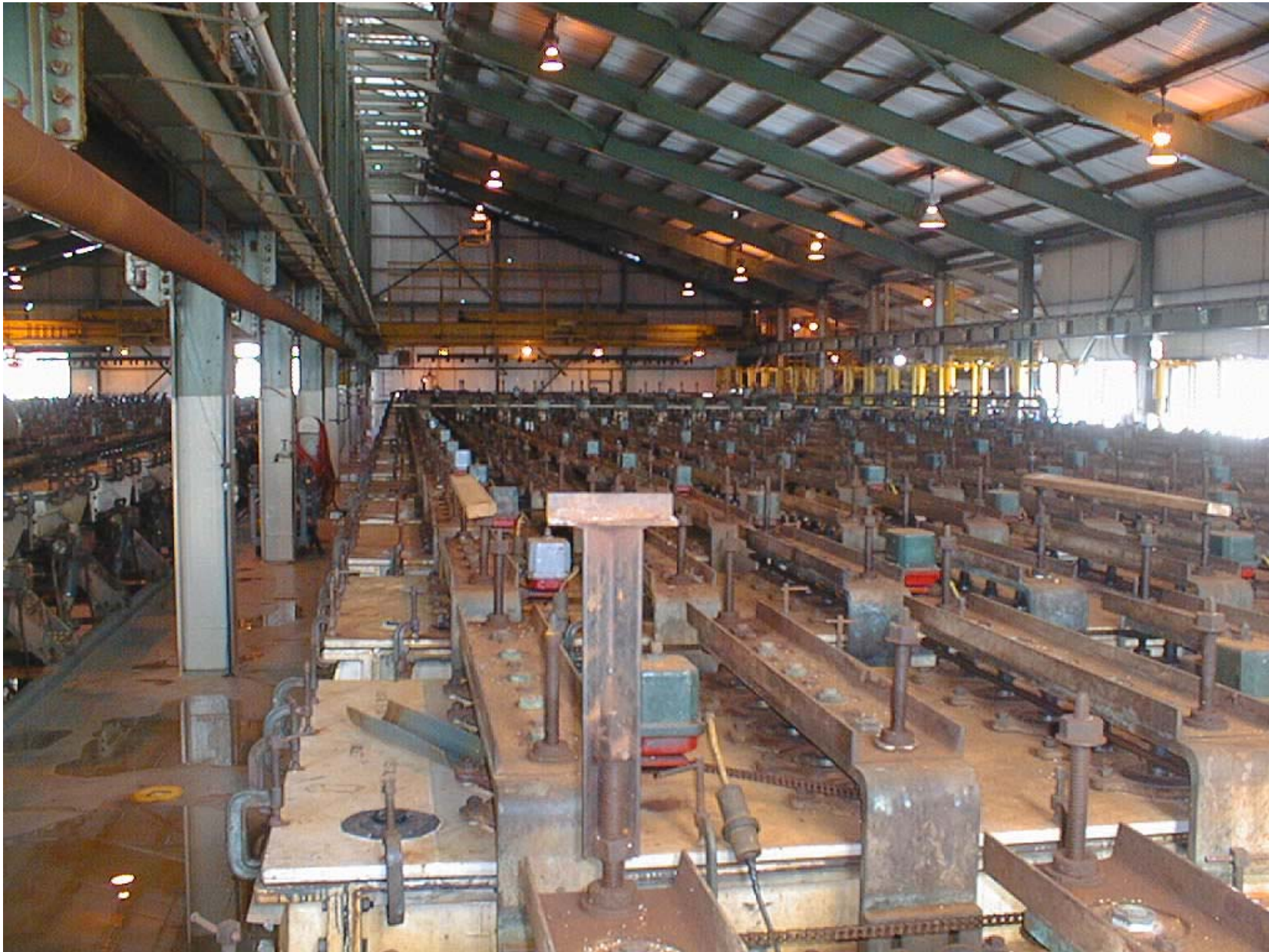
Figure 3-6. North line of electrolytic cells in Olin cell building.
