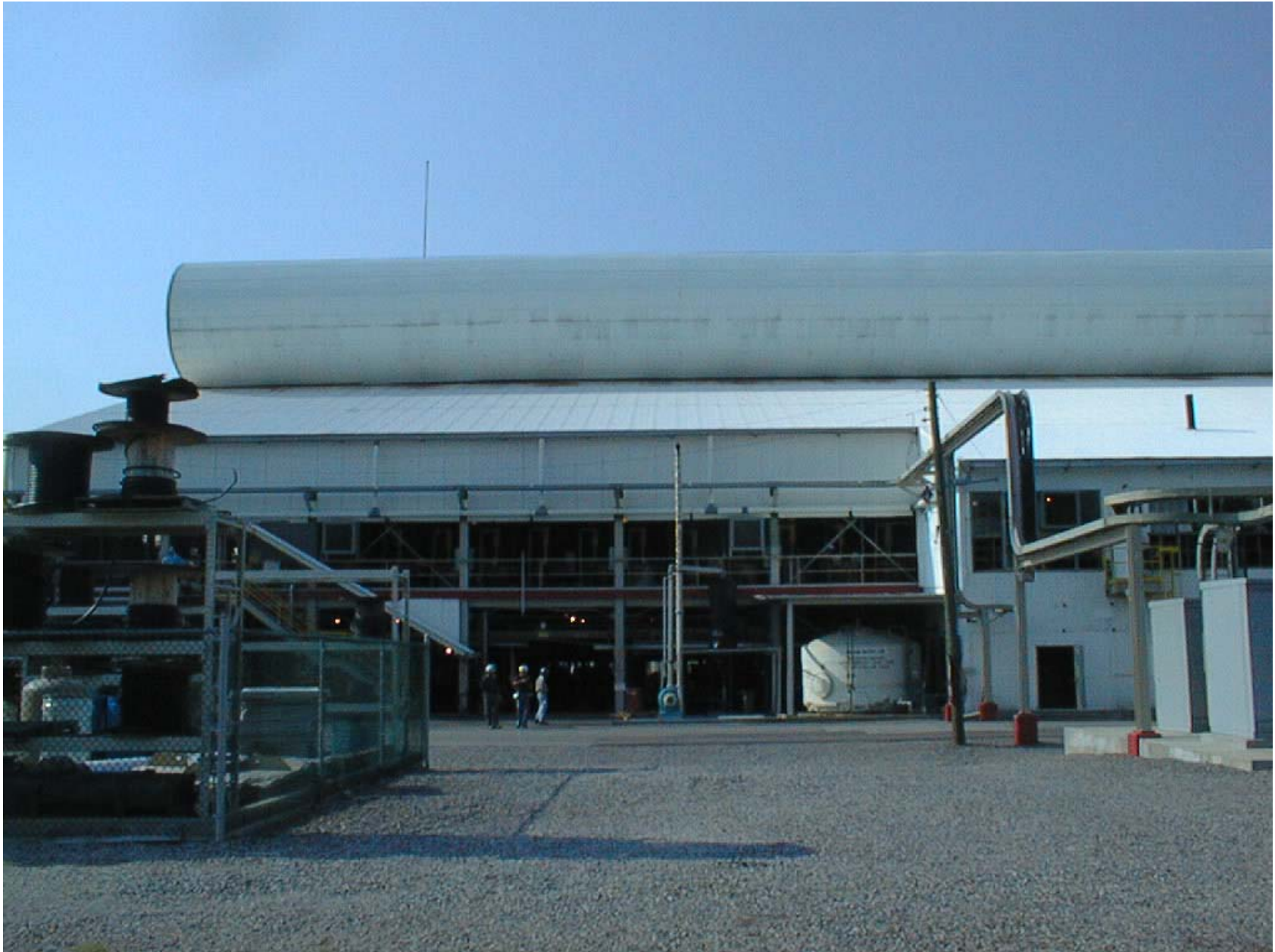
Figure 3-3b. Cell building showing exterior of roof ventilator (from north).
