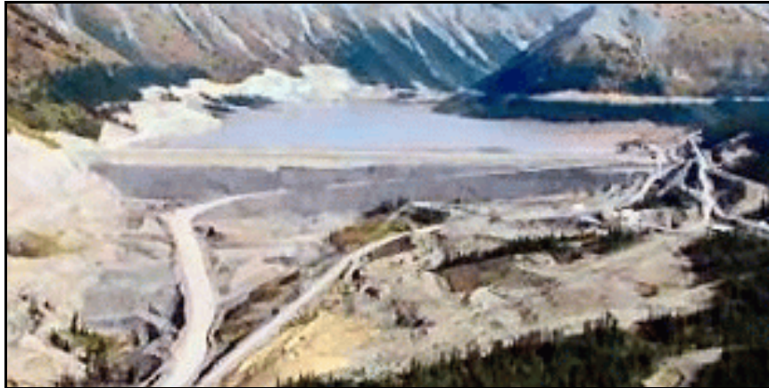
Figure 12. —An example of a tailings dam.
