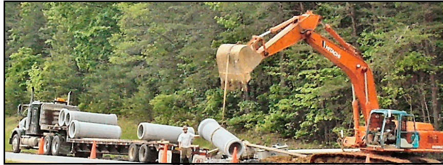
Figure 23. —Precast concrete pipe being unloaded from delivery truck.
