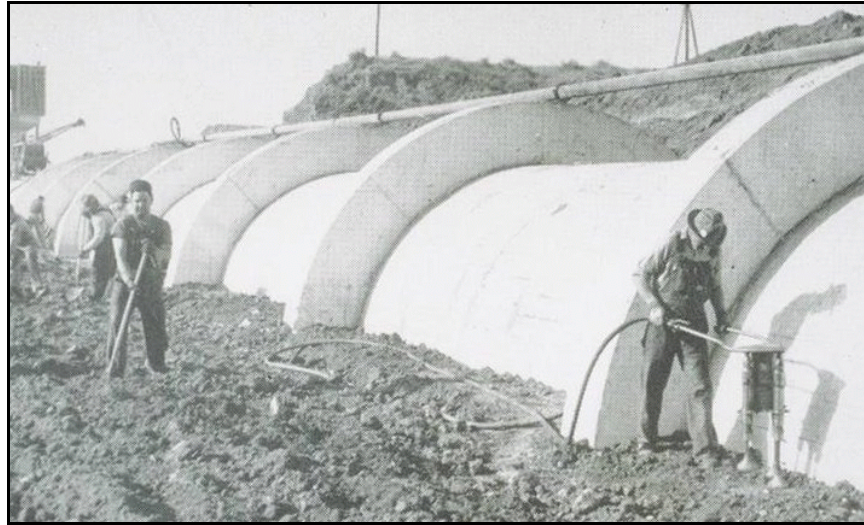
Figure 16. —Good compaction around antiseep collars was difficult to achieve.
