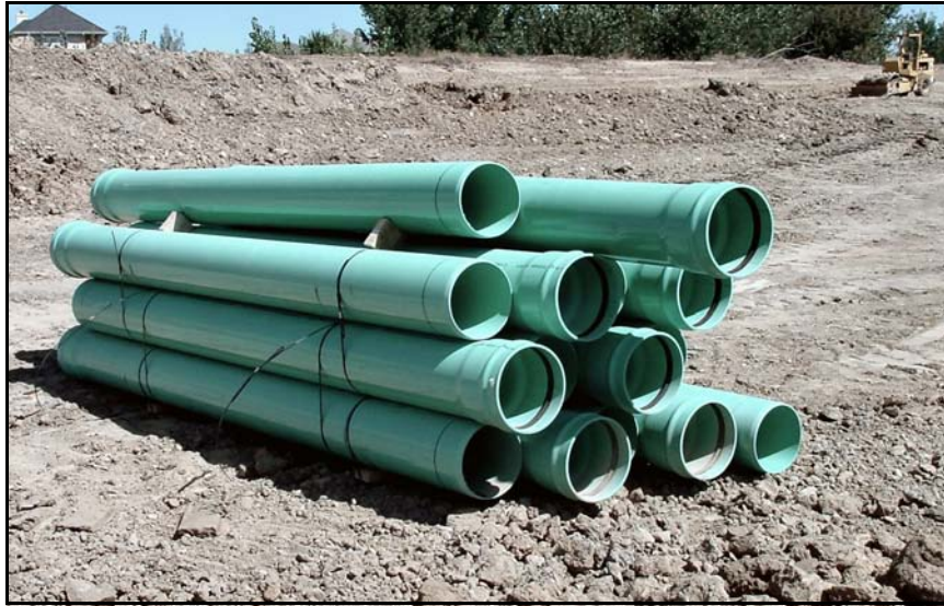
Figure 25. —PVC pipe has infrequently been used in conduit applications within low hazard embankment dams. The bell and spigot joint connection used for this type of pipe limits its use for most conduits.
