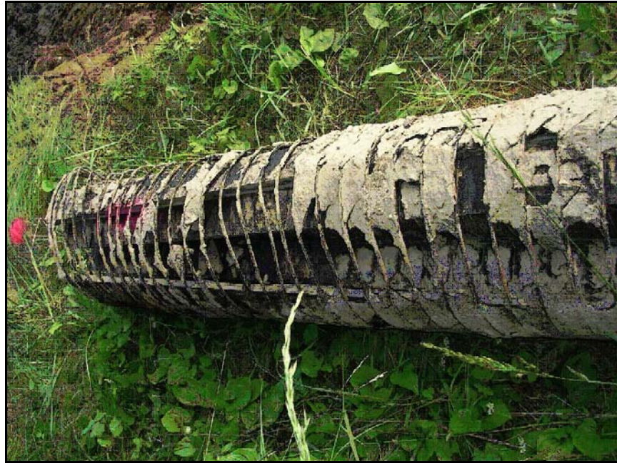
Figure 3. —A 15-inch diameter, wire-wrapped wood stave pipe used as an outlet works conduit within a 75-year old embankment dam. The outlet works conduit was removed and replaced due to deterioration and backward erosion piping concerns.
