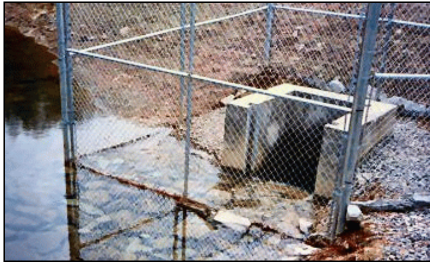
Figure 13. —An example of a decant intake structure.
