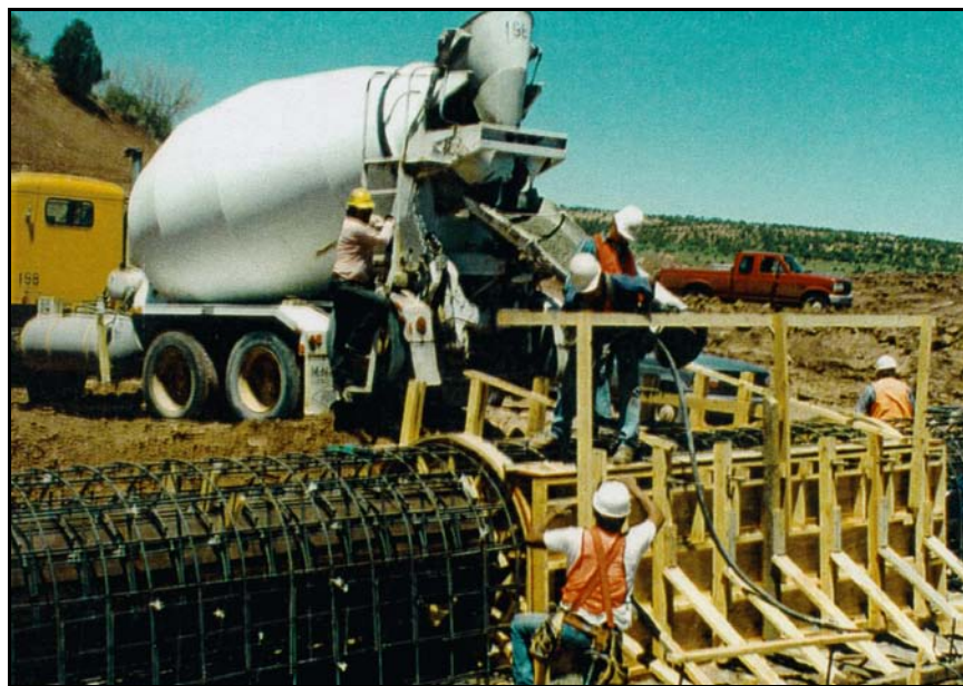
Figure 22. —Concrete placement for a reinforced cast-in-place conduit.
