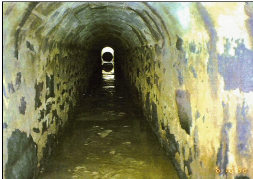
Figure 4. —A 100-year-old, mortar-lined, rubble masonry outlet works conduit.
