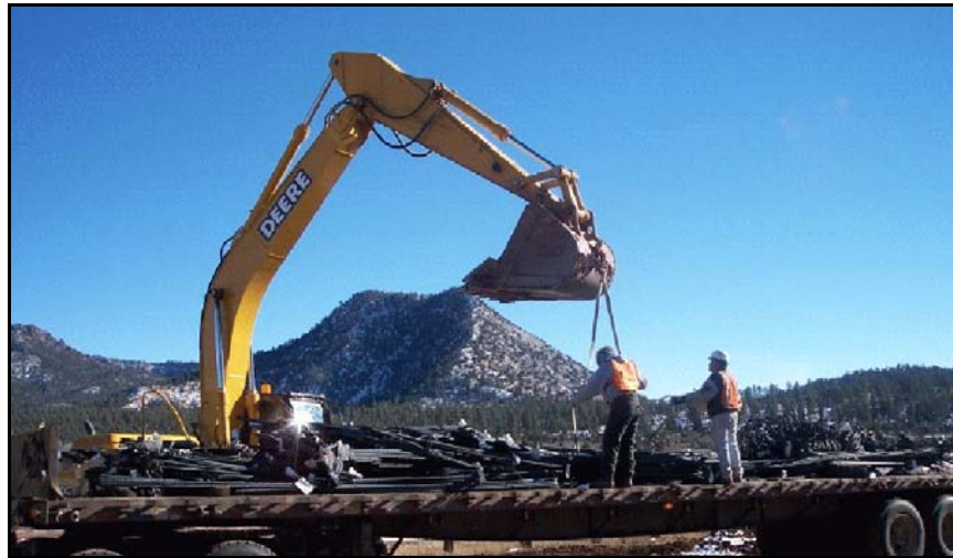
Figure 21. —Reinforcement being unloaded for use in cast-in-place concrete.
