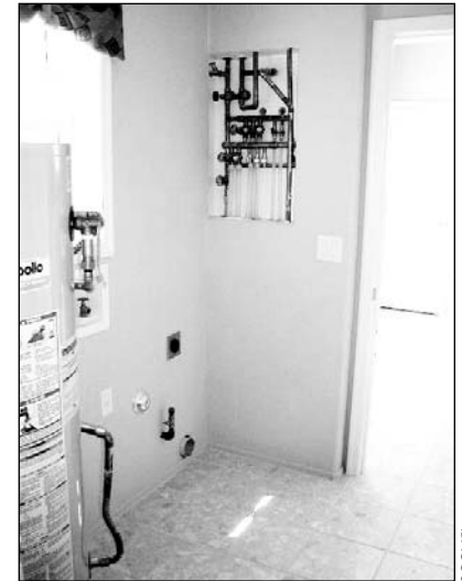
(left) Without instructions, most homeowners didn't understand how to operate the system. (middle) The range limits on this tempering valve on this system were impossible to see, so the homeowners didn't know how to adjust them. (above right) Pre-assembled valve trees save time and reduce problems on site.
