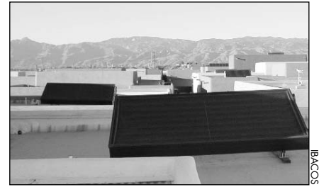
Integral Collector Storage (ICS) panels on Civano homes are part of solar-assisted water heating systems.
