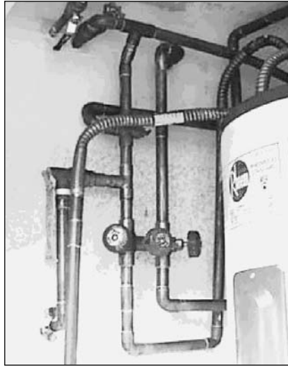
(left) Without instructions, most homeowners didn't understand how to operate the system. (middle) The range limits on this tempering valve on this system were impossible to see, so the homeowners didn't know how to adjust them. (above right) Pre-assembled valve trees save time and reduce problems on site.
