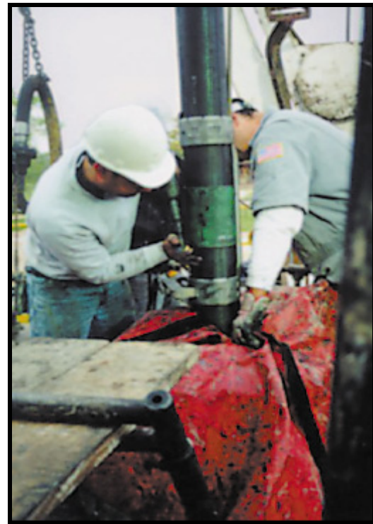
Figure 4: Clamping Wireline on Exterior of the Casing
