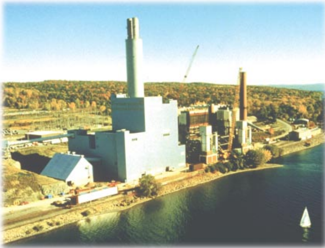
Milliken Station is located in an environmentally sensitive area on the shores of Cayuga Lake, one of the famous Finger Lakes in New York State.
