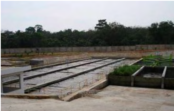
Figure 24 Activated sludge treatment process and experimental beds at PT Jambi Waras Jujuhan
