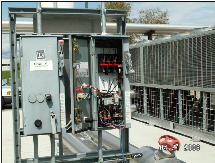
Figure 1.1. 331 Building Chilled Water Pump #2 Electrical Panel
