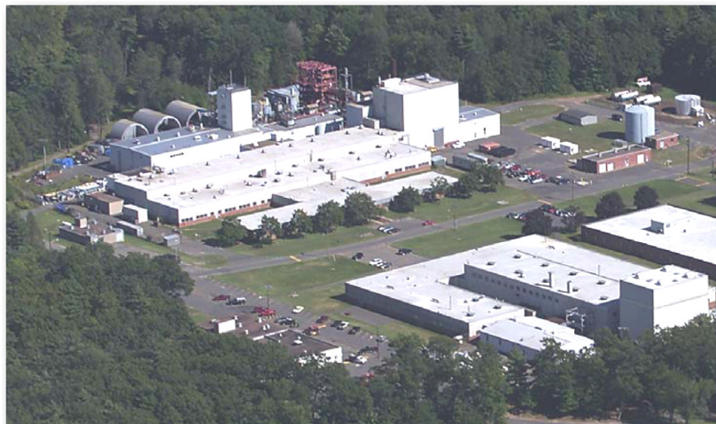
ALSTOM Power Plant Laboratories
