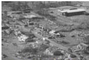
View of tornado's destruction. Photograph courtesy of Dewitt Era Enterprise Newspaper
