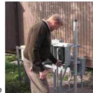
Allen Hansen works on an electrical panel. Photo by Chuck Ryan.
