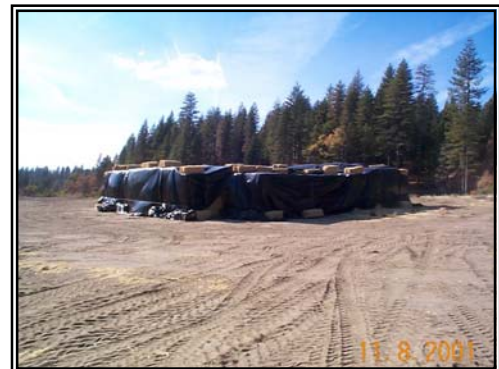
Staging Area with Straw
