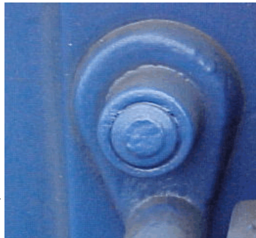
Typical two-part mechanical fastener
