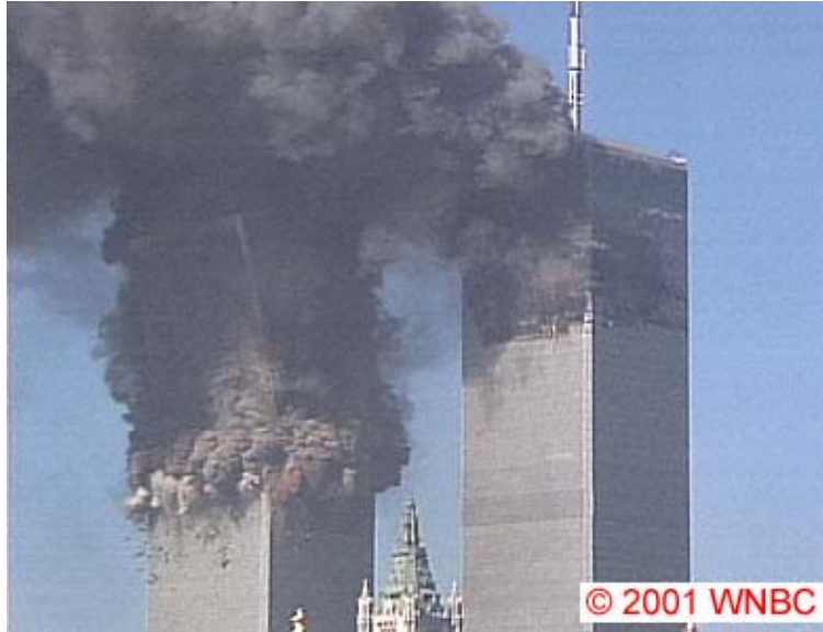
Figure E–8. View of upper building section of WTC 2 tilting to the east.
