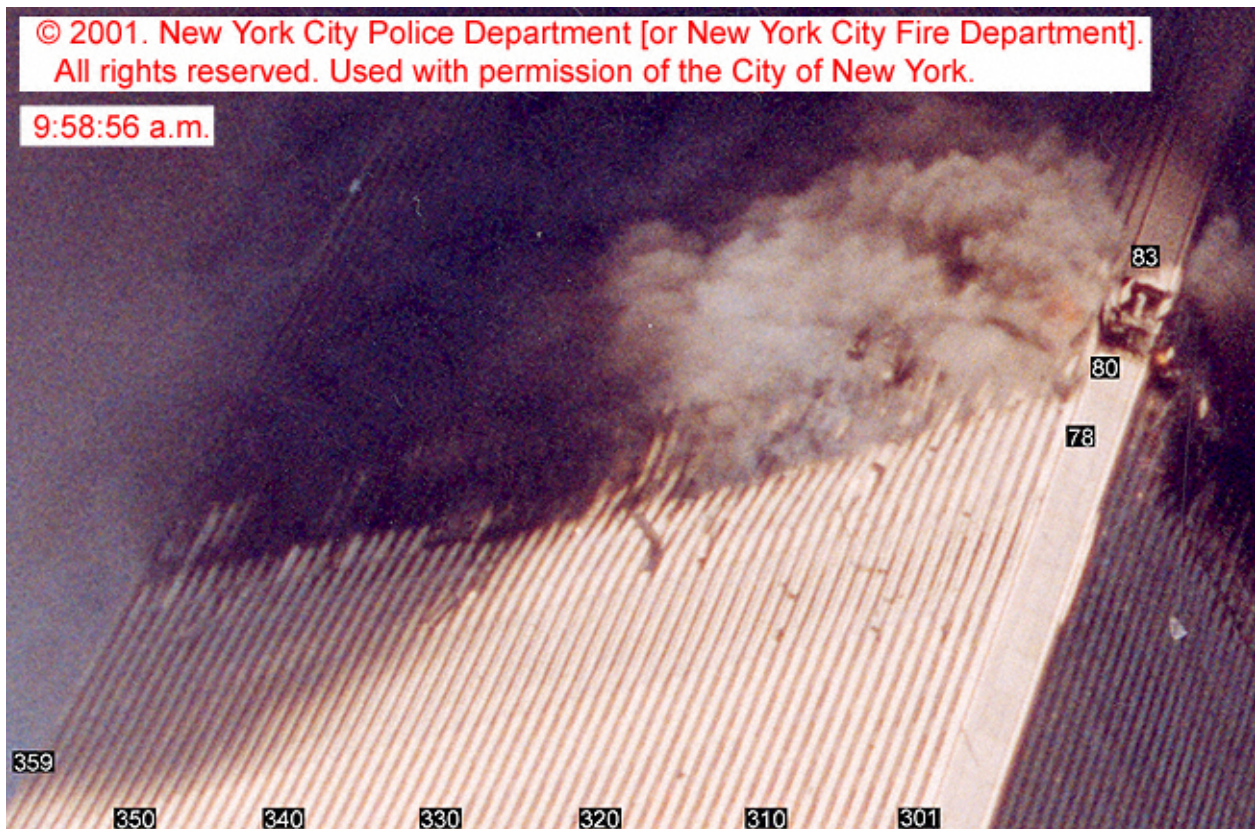
Figure E-7. View of WTC 2 buckling of east wall near northeast corner as collapse initiates from southeast.
