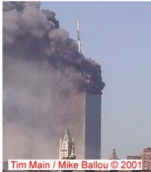
Figure E-6. WTC 1 building section above impact damage zone tilts to the south.
