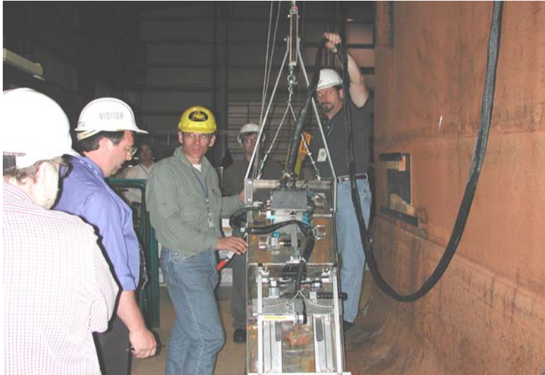
Figure 8.1. RONDE Deployment Platform
