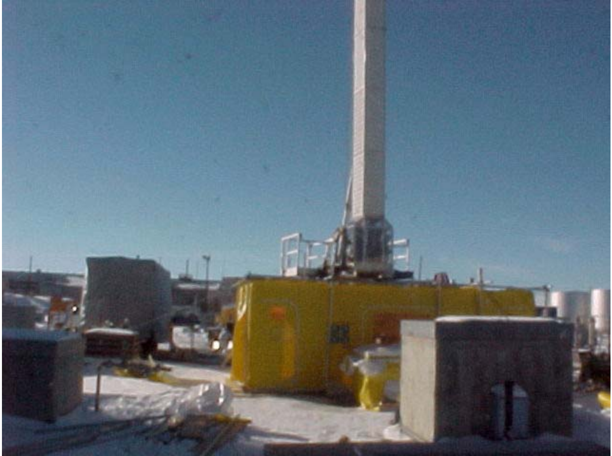
Figure 1. LDUA Deployed over Tank WM-188.
