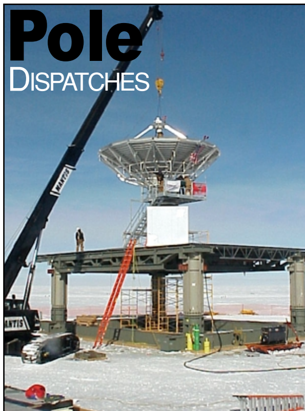
The MARISAT/GOES satellite dish was recently placed at South Pole Station. The dish will allow Pole to be in constant communication with the rest of the world. The station now goes through daily blackout periods when the satellites it uses for internet and phone communications dip out of view. Photo by Jerry Macala.
