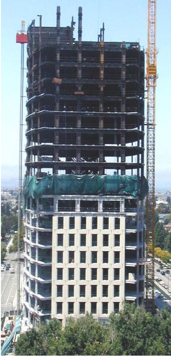
a. Building above is a high-rise steel dual system – moment frame (heavy columns and beams on upper facade) with bracing around elevator core. Fireproofing is being applied to steel at mid-height (inside the shroud) and precast facade elements are being attached to frame in lower stories.
