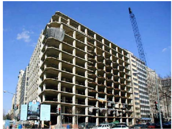
c. New precast facade units being applied to reinforced concrete frame buildings.
