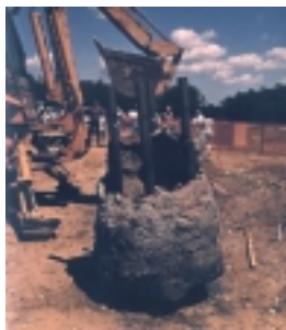
Following in-situ vitrification, a solid block of glass remains after cooling.
