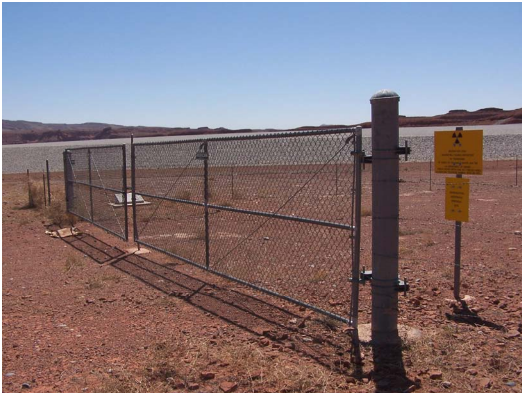
HAT 4/2006. PL-1. Entrance gate (showing bent center rod) and sign, site marker; disposal cell in the background.
