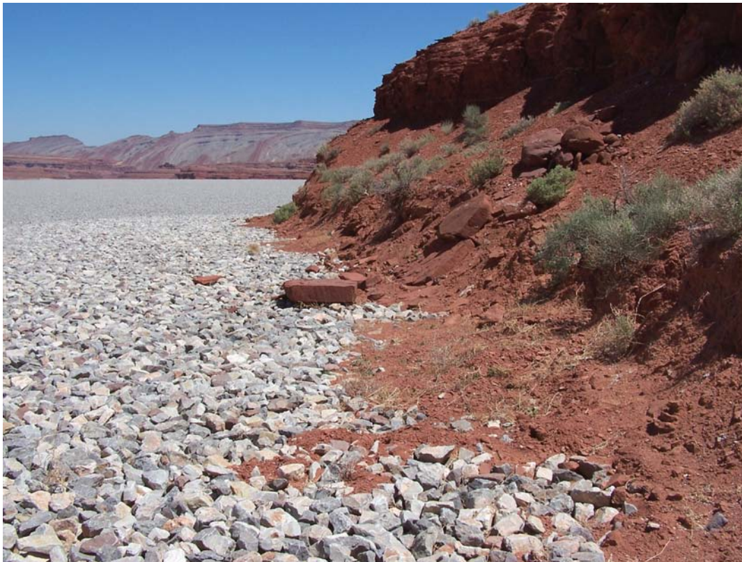
HAT 4/2006. PL-3. View northeast along the southeast apron showing insignificant accumulation of detritus.
