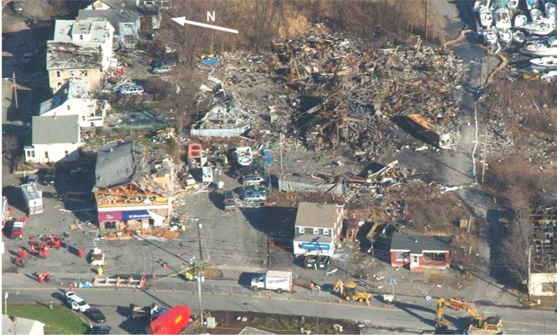
Figure 10. Aerial view of CAI/Arnel facility after explosion and fire (bakery/pizzeria building lower left) (ATF photo).
