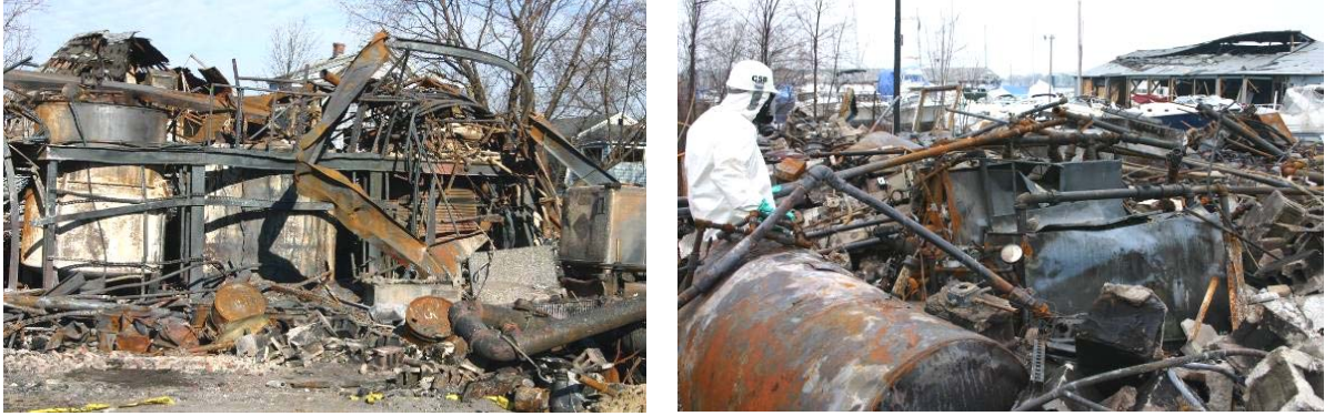
Figure 16. Explosion and fire destroyed the CAI/Arnel building.
