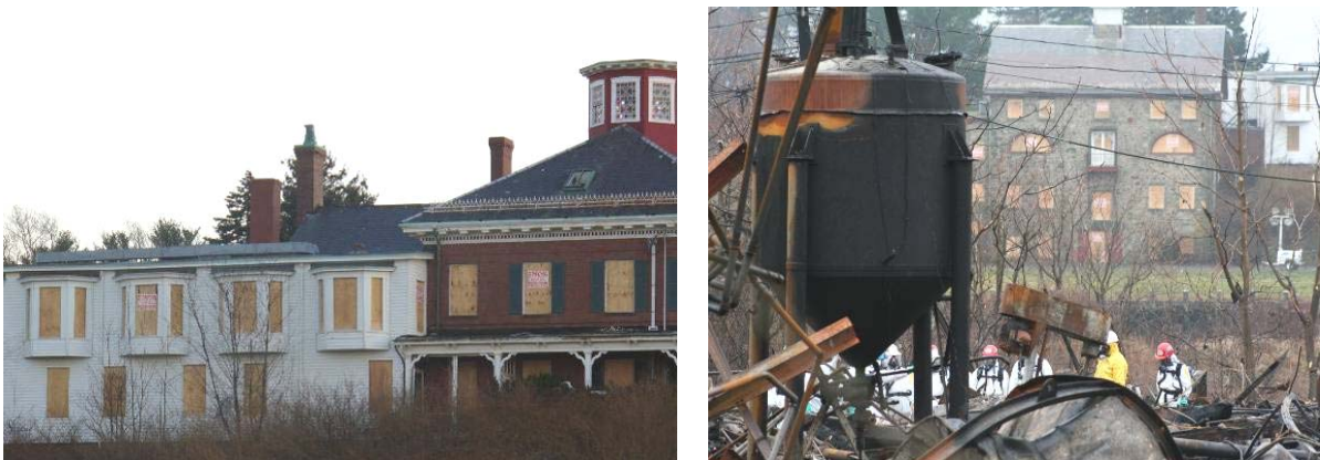
Figure 13. Shattered windows and doors boarded up at the New England Home for the Deaf, 800 feet from the explosion.
