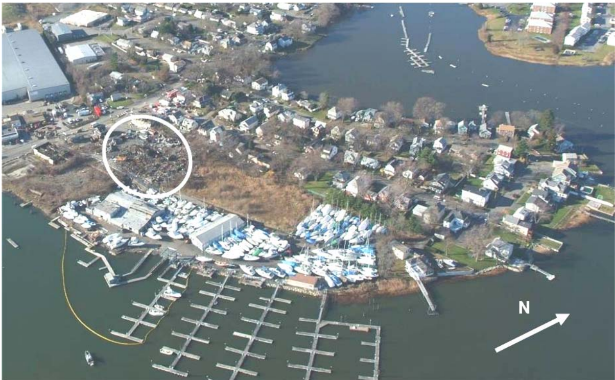
Figure 1. Danversport peninsula. CAI/Arnel facility explosion site circled (ATF photo).
