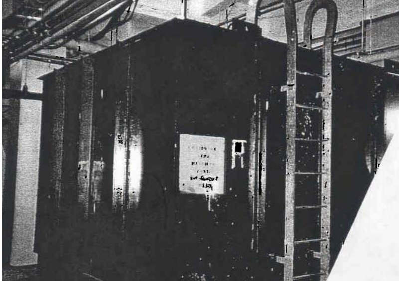
Figure 3–3. Typical 5,000 gal water storage tank, WTC 1 and WTC 2.
