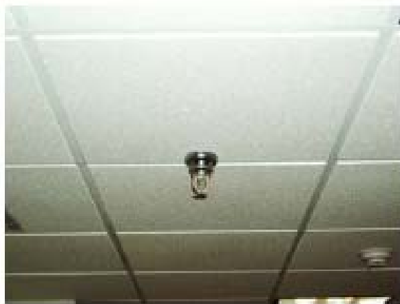
Figure 3–1. Typical sprinkler installed in ceiling.
