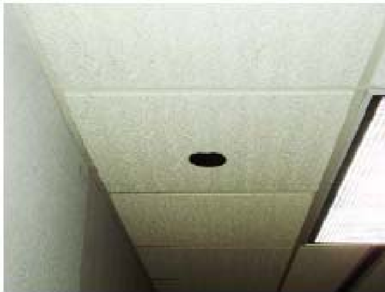
Figure 3–7. Typical concealed pendent sprinkler.
