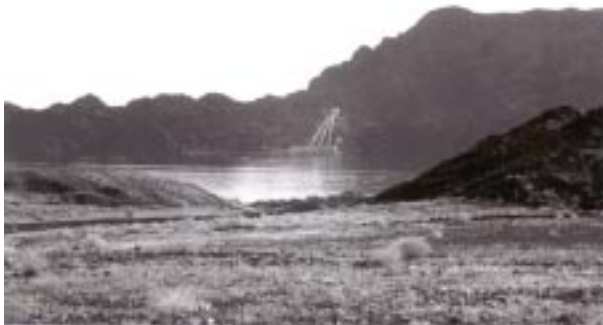
Fig. 37. Metropolitan Water District's pumping plant on Lake Havasu.
