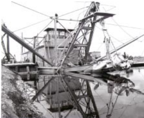
Fig. 23. The dredge Colorado straightened 30 miles of the Colorado River near Needles, California. Here the dredge is tied at Needles in 1949, P423-3000-1808A. Courtesy of the Bureau of Reclamation, Boulder City, Nevada.
