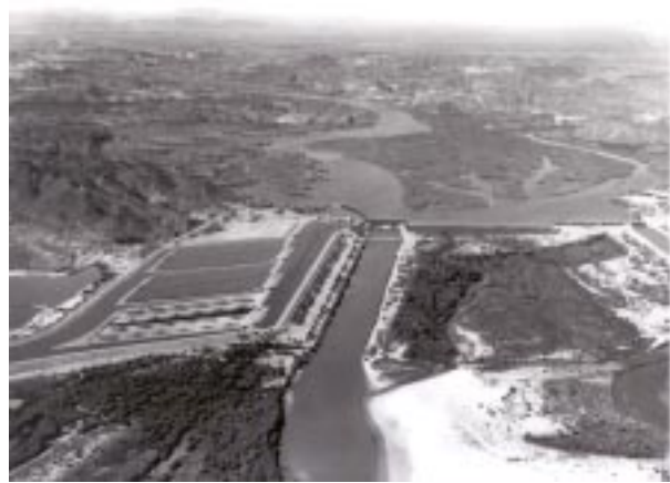
Fig. 30. Imperial Dam, P212-3000-3890-1A. Courtesy of the Bureau of Reclamation, Boulder City, Nevada.
