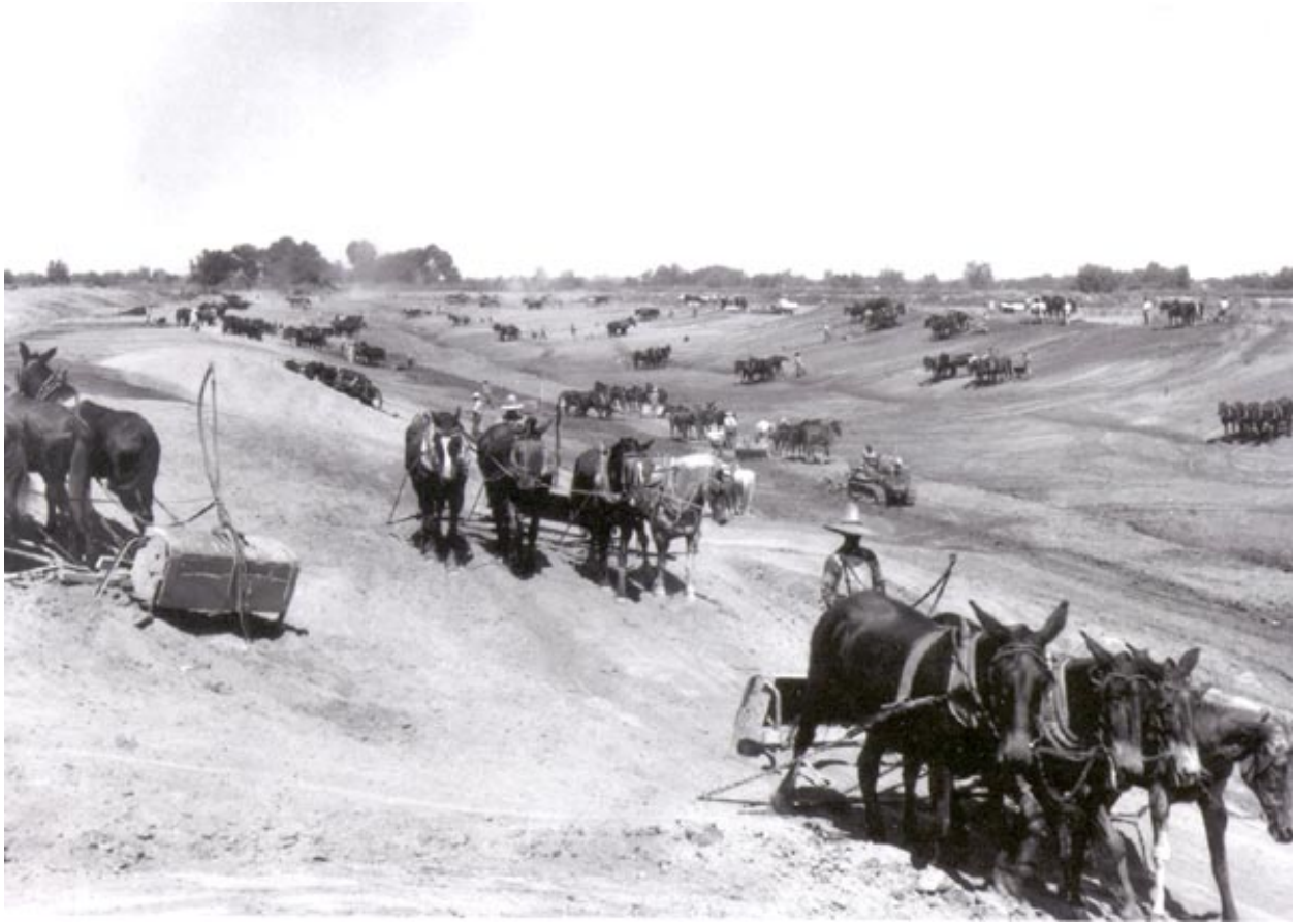
Fig. 22. Horse and mule-drawn scrapers help dig the All-American Canal in 1935, P212-303-269A. Courtesy of the Bureau of Reclamation, Boulder City, Nevada.
