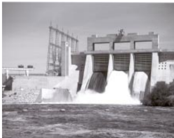
Fig. 32. Davis Dam. Courtesy of the Bureau of Reclamation, Boulder City, Nevada.
