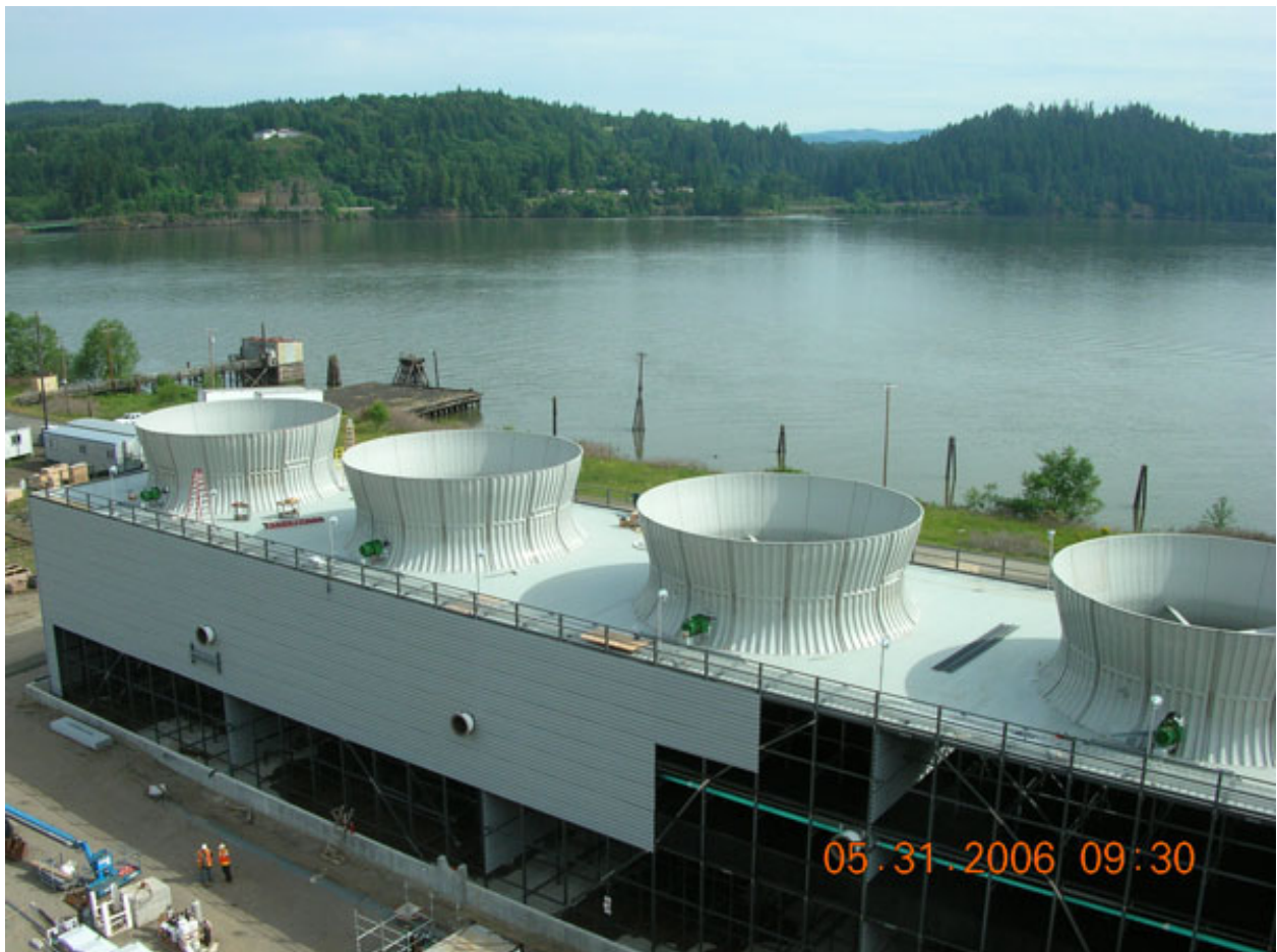
Figure 8. Example of forced convection cooling towers.
