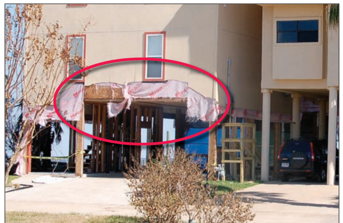
Figure 3. NFIP-compliant breakaway wall construction.
