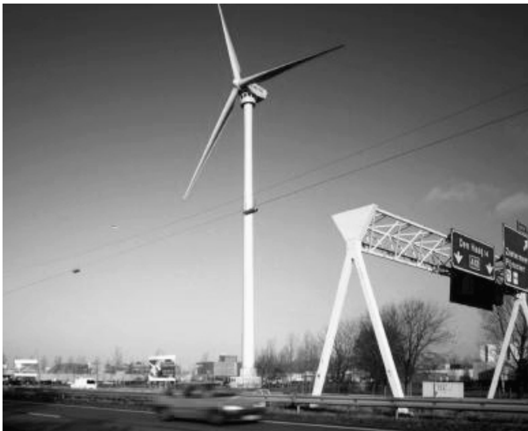
Figure 18.4 Enron-Tacke 1.5 MW with rotor 70.5 m with view platform just under the nacelle
