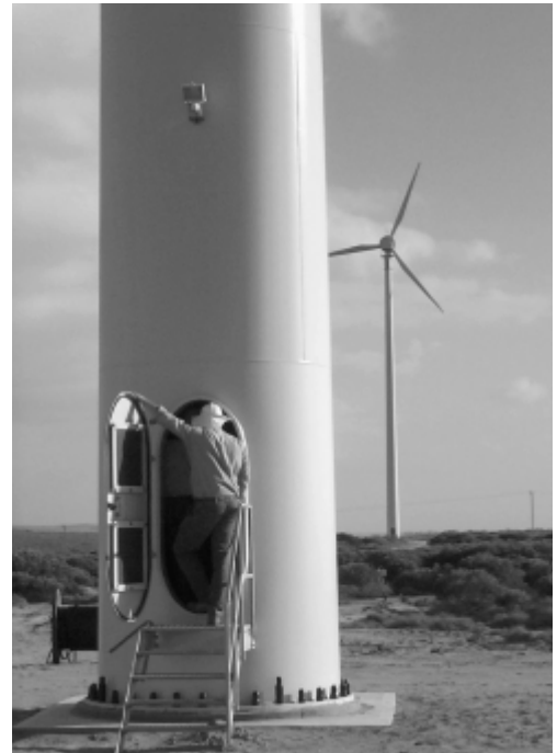
Figure 9.6 Denham wind-diesel power system with flywheel storage, Western Australia
