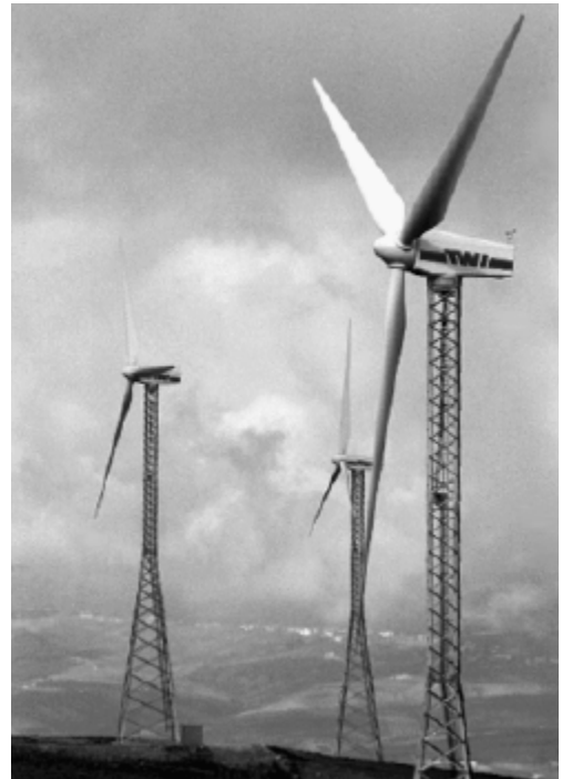
Figure 15.5 IVPC 4 27 MW windfarm at Bisaccia (12 wind turbines Vestas IWT 600 kW and 30 IWT 66 kW)
