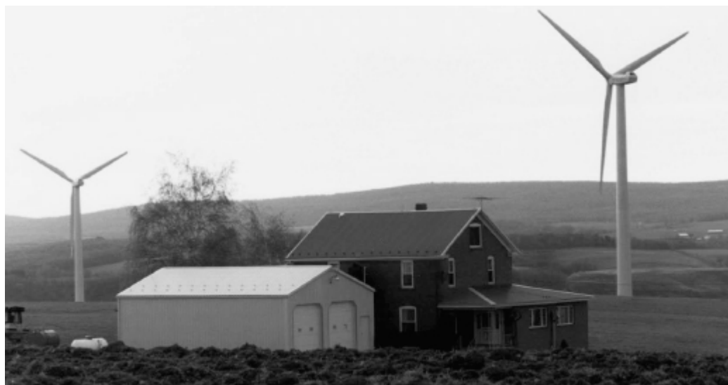
Figure 23.2 The 10-MW wind power plant located in Garrett County, Pennsylvania
