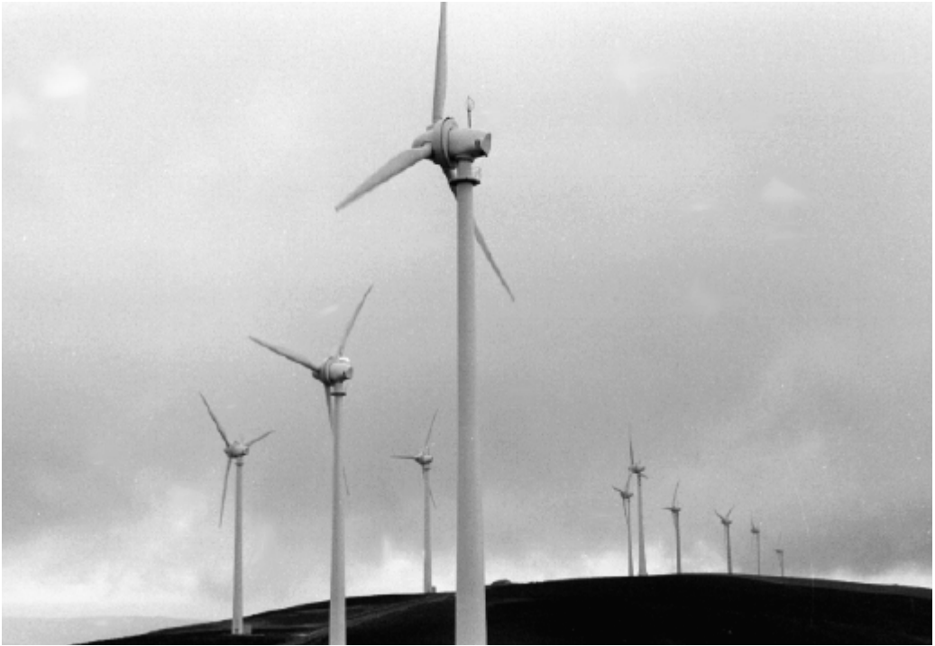
Figure 15.4 Edison Energie Speciali 10 MW windfarm at S. Giorgio la Molarra (20 wind turbines Enercon 500 kW)
