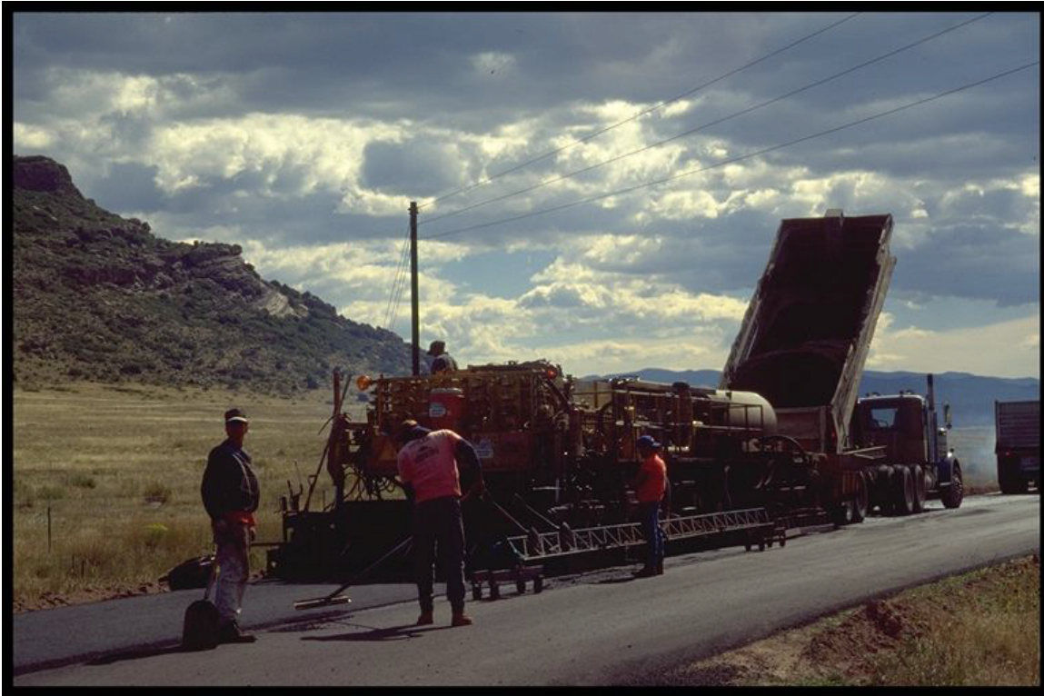
Figure 9-5. Repaving process.
