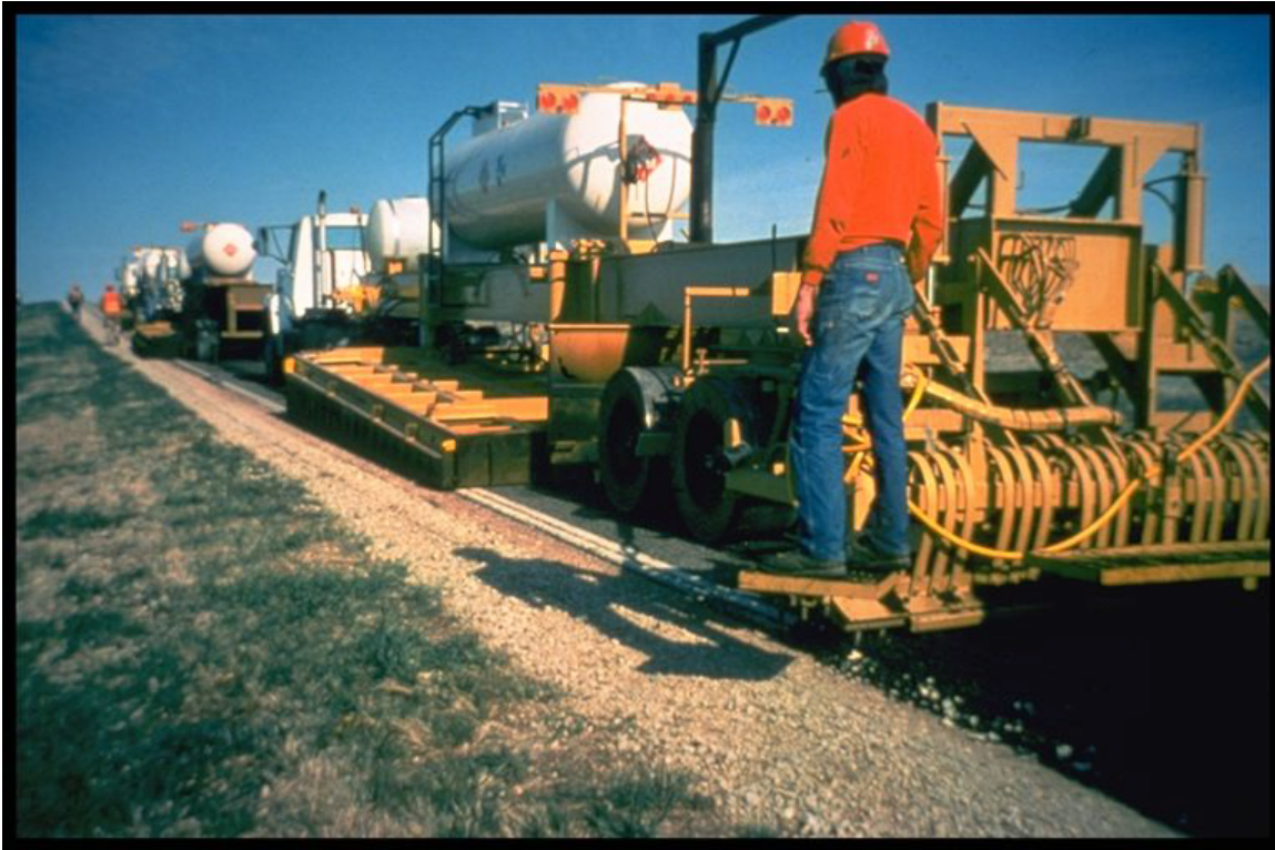
Figure 9-2. Surface recycling.
