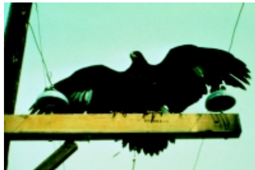
Figure 50.2 This is a hazardous situation because the eagle's wings can contact two conductors at once.
