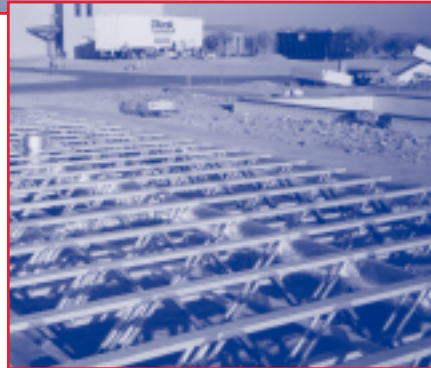
Heating and cooling ducts are routed through open-web floor joists in a sealed crawl space for this Building America house in the Civano Community in Tucson, Arizona .
