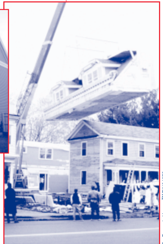
A third-story module is lifted into place on a prototype Building America duplex in a Cambridge, Massachusetts infill project. Epoch Corporation is the modular builder partner.
