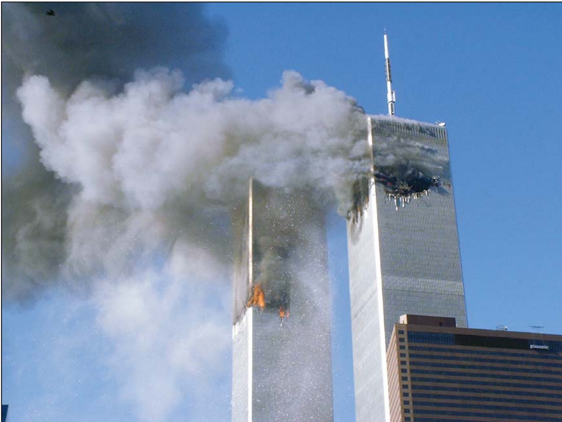
Figure 1-6 View of the north and east faces showing fire and impact damage to both towers.
