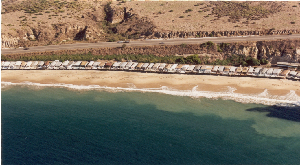
Figure D.4.6-20. Sand Beach Backed by Shore Protection Structures, Crystal Cove, California (Source: Noble Consultants)
