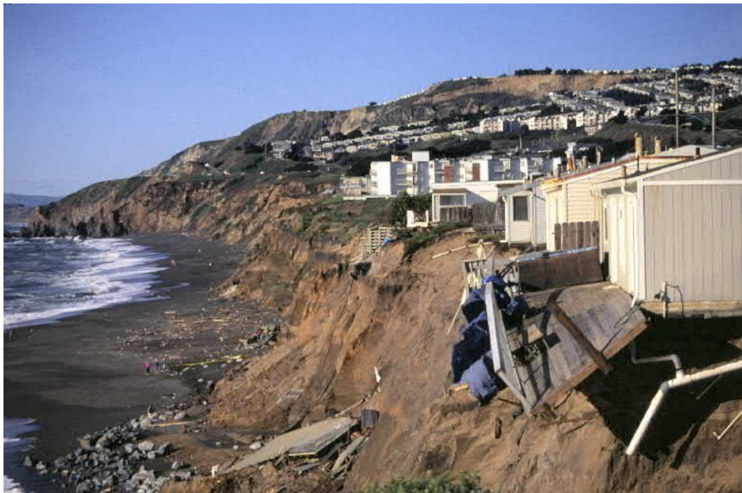
Figure D.4.6-28. Bluff Failure and Retreat During 1998 El Niño Storms, Pacifica, California (Photo by Kevin Coulton)
