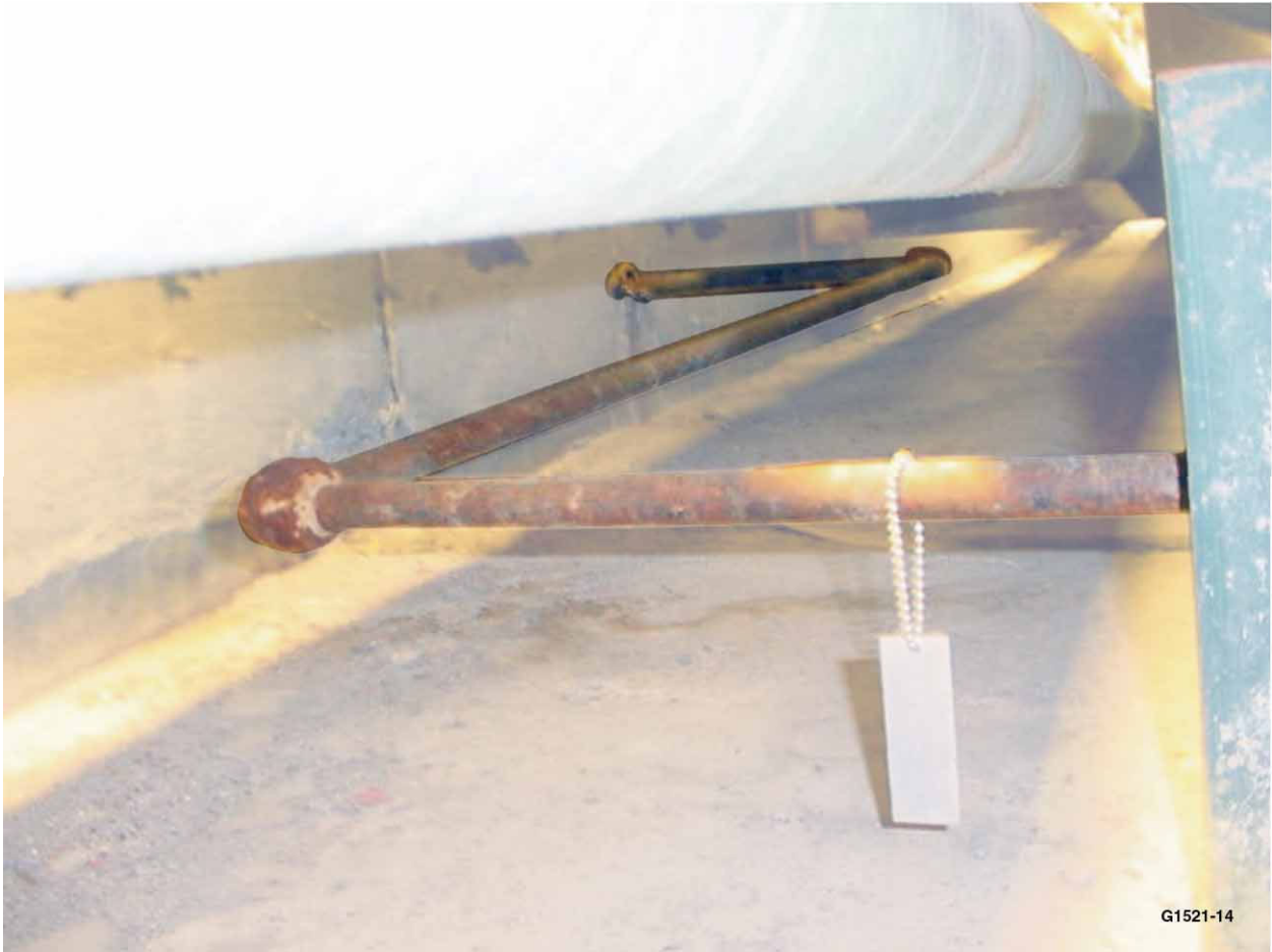
Figure 16. Photograph of the drip leg inside the utility tunnel (from DOE/NE-ID 2004).
