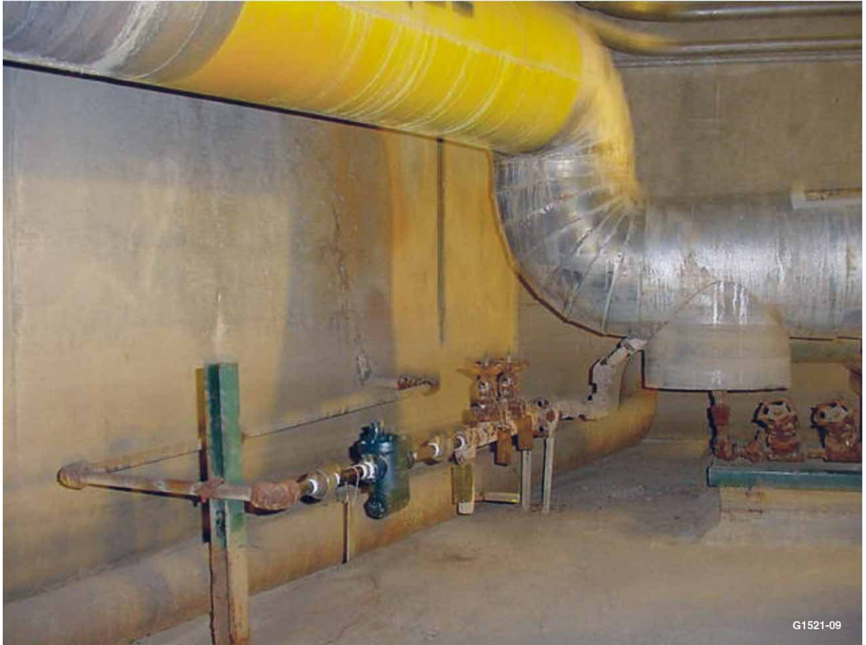
Figure 11. Photograph of the drip leg inside the utility tunnel (from DOE/NE-ID 2004).
