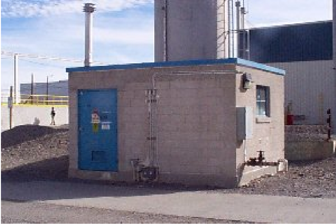
Figure 4. Photograph of building CPP-702 prior to demolition (from ICP 2005).
