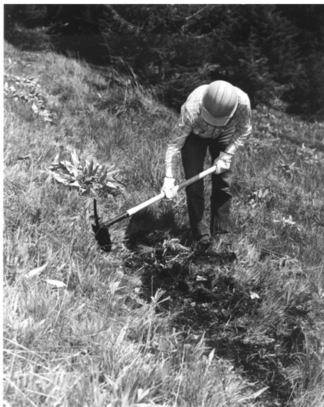
Combination (or Combi) tool developed for firefighting, is popular for trail work.
