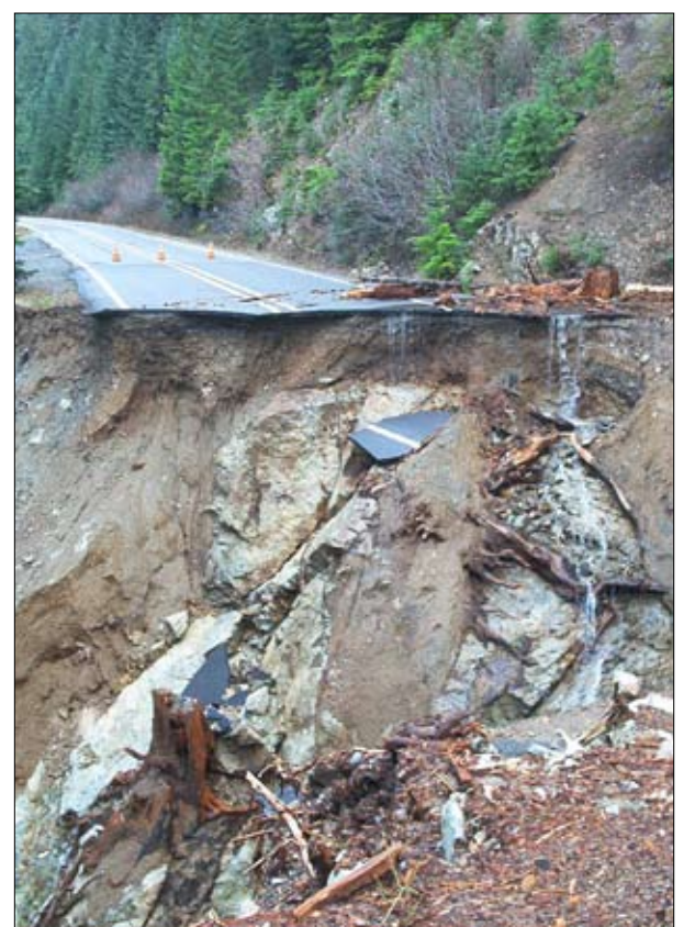
One of four washouts on Highway 123, between Ohanapecosh and White River.
