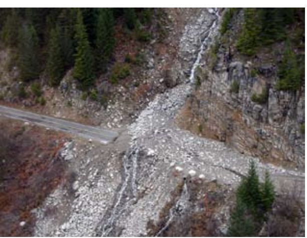
A landslide on Steven's Canyon Road.
