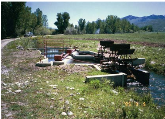
Photo 2.3-4. New fish screen in Lemhi Subbasin.
