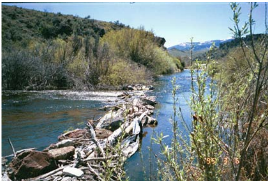
Photo 2.3-2. Push-up dam on Lemhi River.
