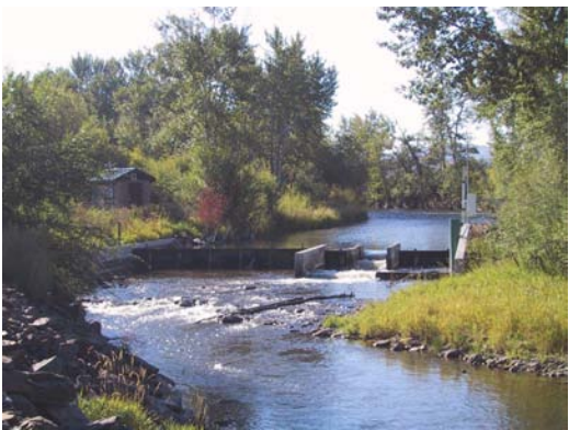
Photo 2.3-1. L6 Diversion structure on the Lemhi River.
