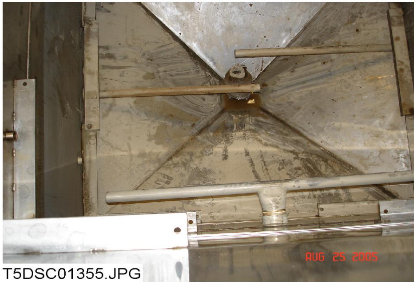
Figure 3-93. Tank bottom after draining.
